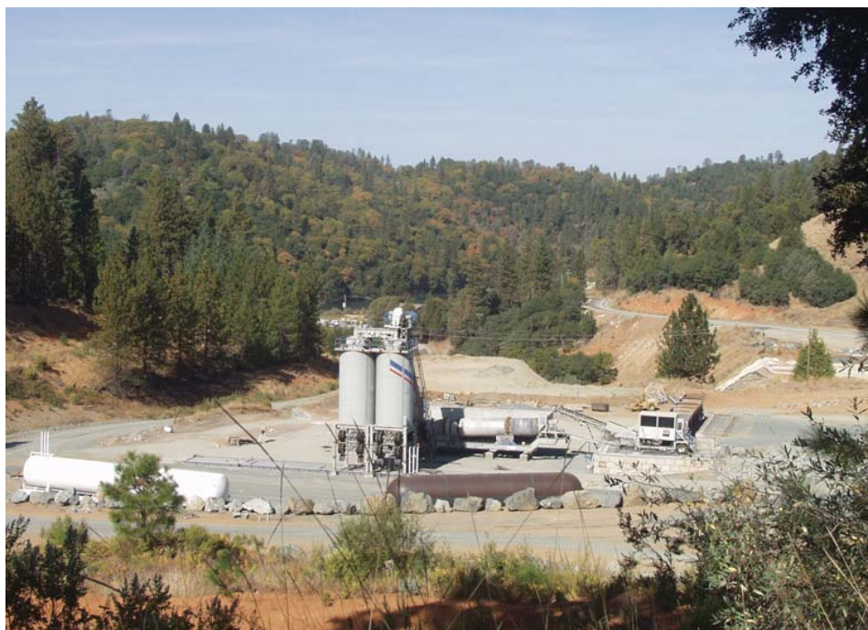
Chevreaux Aggregates Meadow Vista Asphalt Plant 10/26/06
