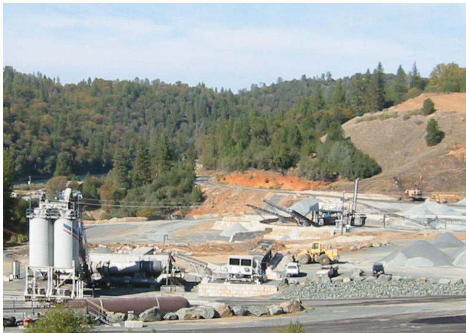
Chevreux Aggregates Meadow Vista Asphalt Plant 10/26/07
